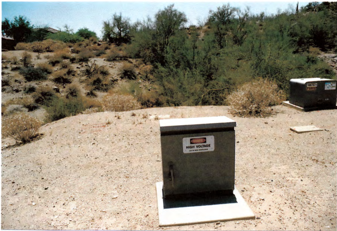
Photograph #3- View of drainage way located along west Site vicinity-
